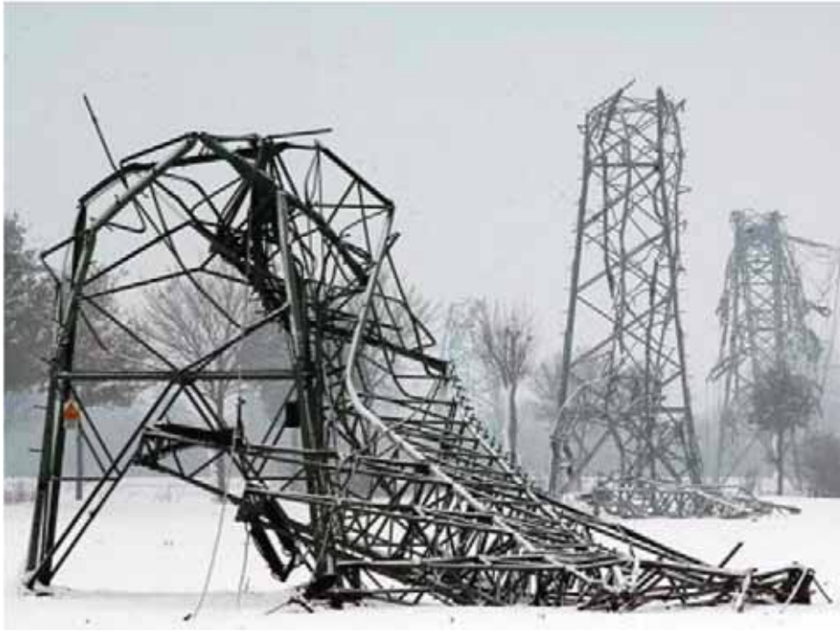
Figure 3.2. Extreme Ice and Snow Loads on Pylons Near Münster, Germany, in Autumn 2005
